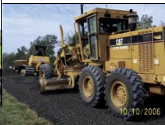
Levee Board spreading limestone.
