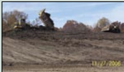
488L - Topping out the levee.
