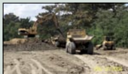
488L - Loading dump trucks with dike material.
