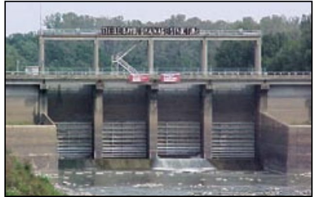
Steele Bayou Drainage Structure
