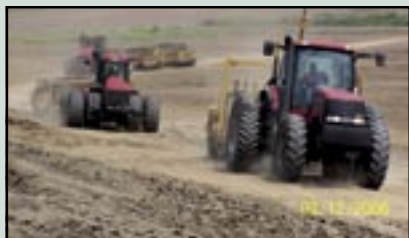
488L - Enlarging levee base.
